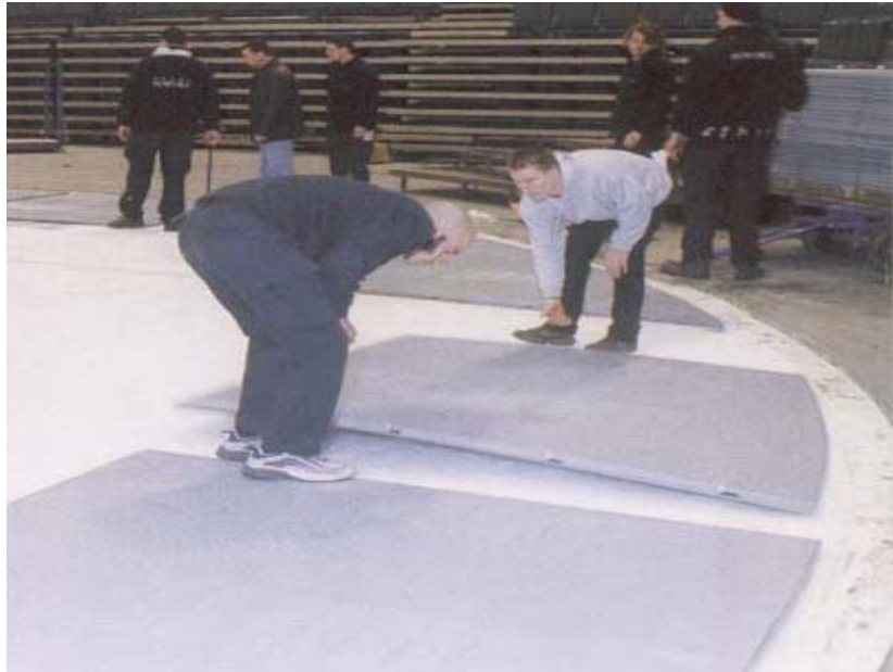
Positioning the pre-cut corner Tiles.
