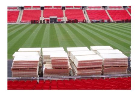
4.2 Trolleys should be provided to keep movement of blocks by hand to a minimum. A full pallet should be loaded onto each trolley at the edge of the field by forklift.
